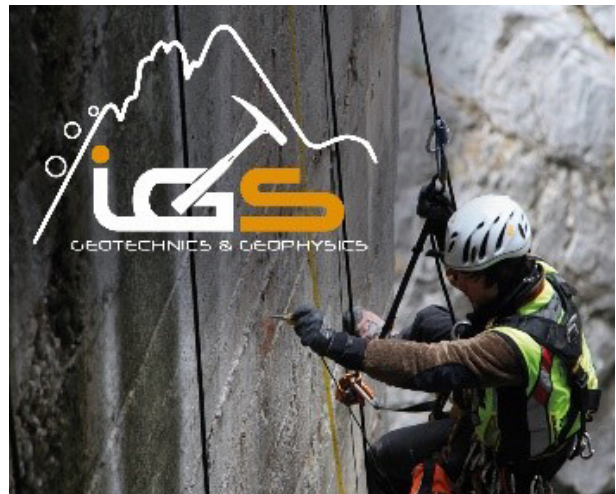
IGS executing on-the-wall surveys, 200m from the ground
